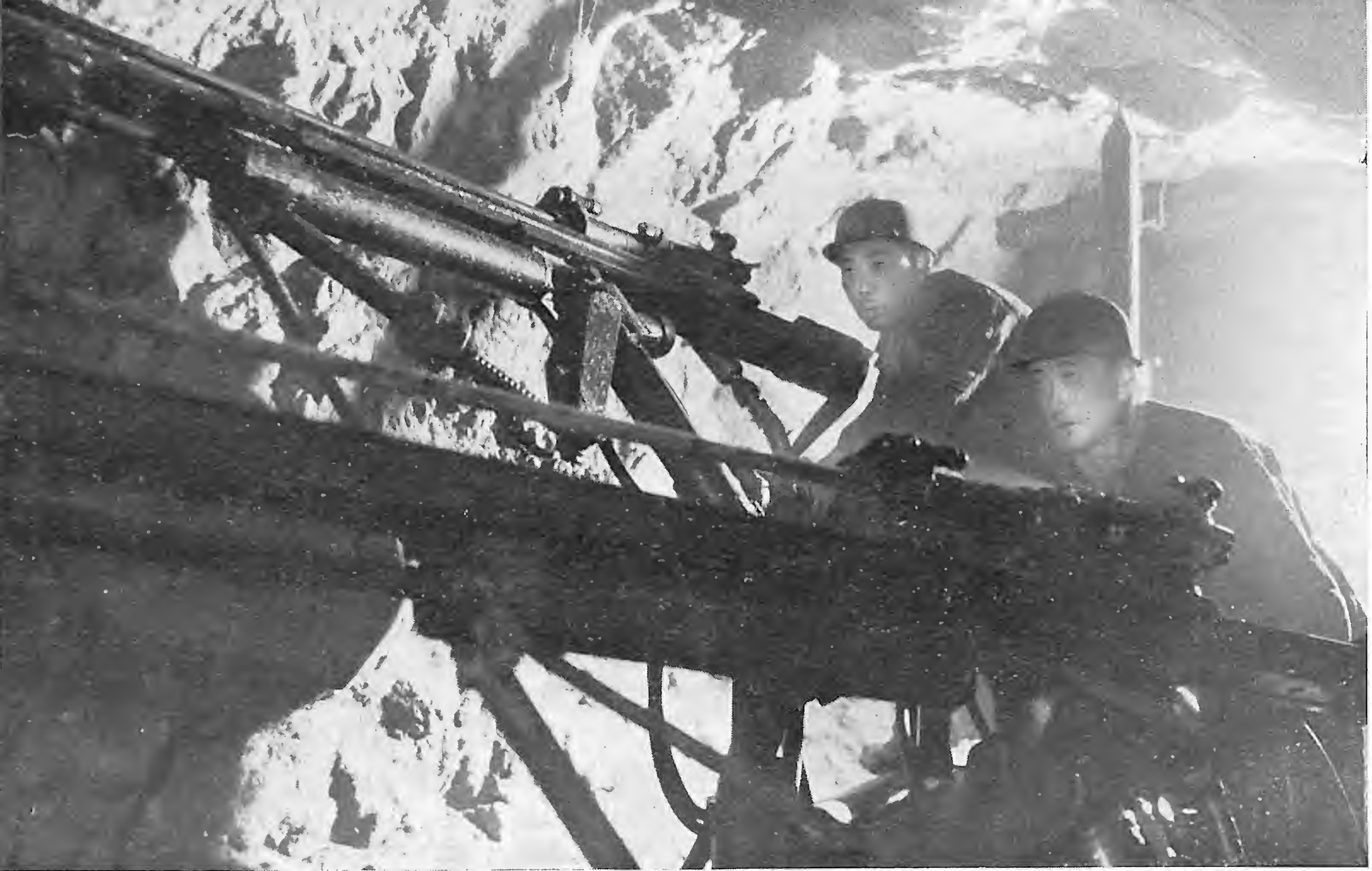
Twin-boom hydraulic drill car in operation.
